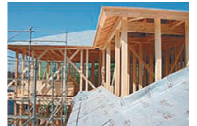
Breathable heat shield roofing sheet under roof tile
